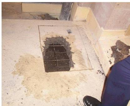
**Fig 4. Hole in concrete floor, to destroy termites found with thermal imaging.**
