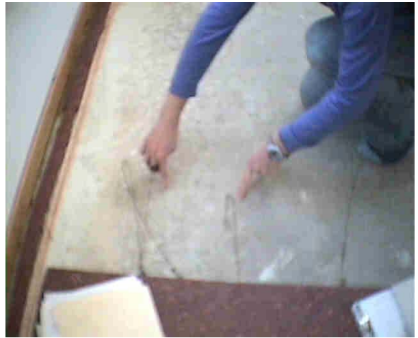
Figure 7. Radiant tubing locations identified in basement slab for purposes of slab coring and soil testing.
