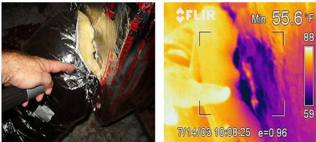
Figure 8. Supply junction of flex duct and disbursement box that was not sealed or taped
