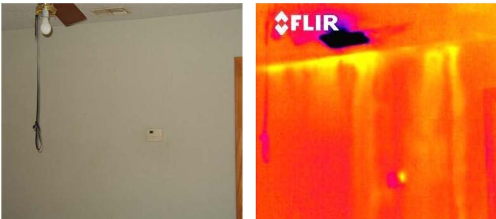
*Figure 4. Thermal ducting inside a hollow wall behind the thermostat*
