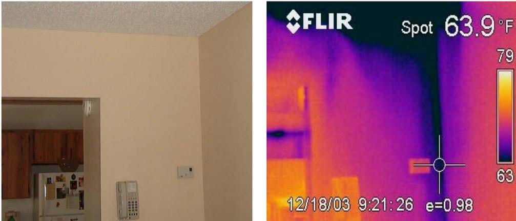
*Figure 5. Cold air being drafted in a hollow wall behind the thermostat*
