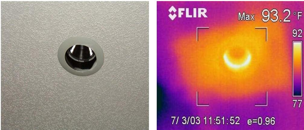
*Figure 3. Ceiling penetration and insulation problem*
